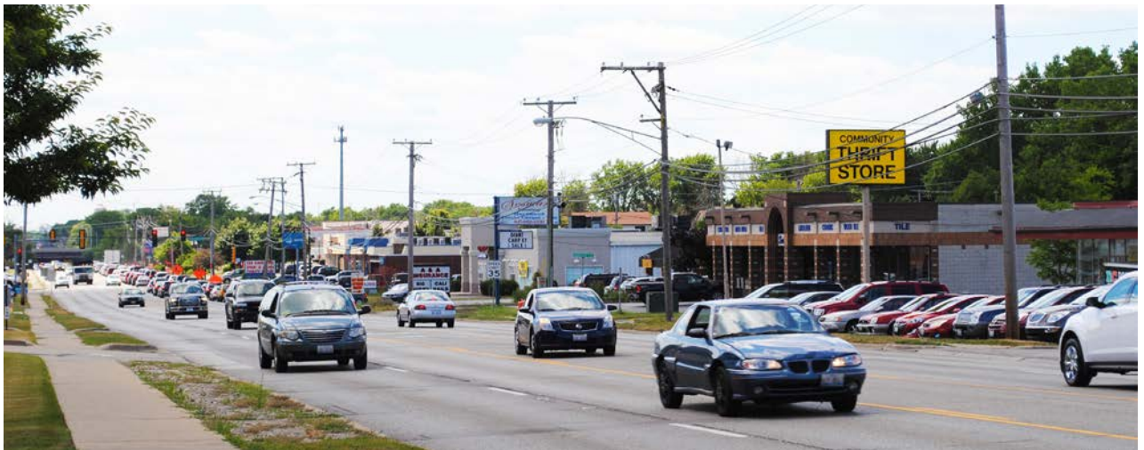
East Grand Avenue Study Corridor: view looking west and aerial map.
